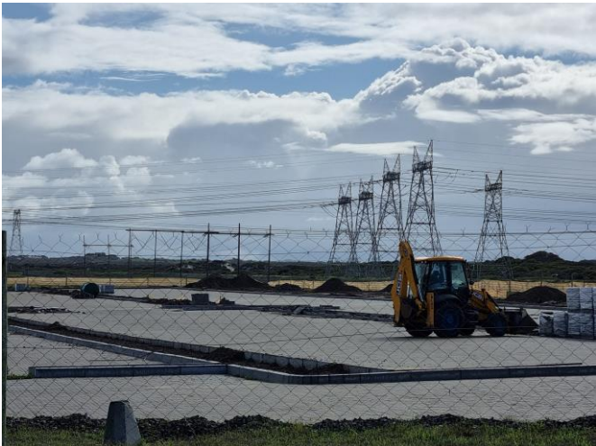
Image 10: Parked plant and neat working area
