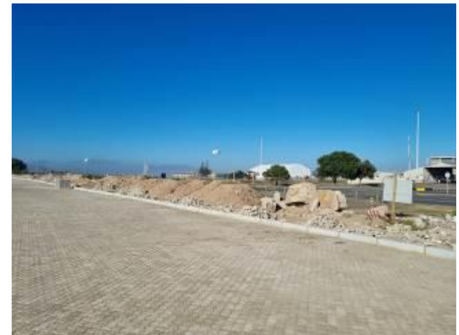
Image 6: Storage of aggregate on site.
