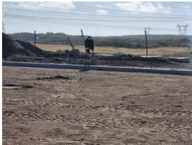
Image 5: Cleared area awaiting paving.
