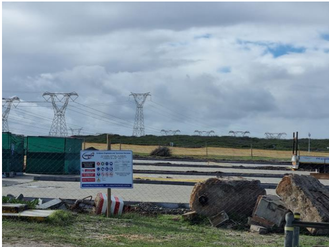
Image 9: Site Camp and working area
